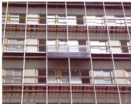
**Fig 6:** two-shelled external wall of Supreme Audit Court Building.
