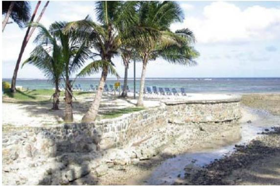
Fig. 3 Erosion of shoreline and damage to tourism infrastructure due to hurricane IVAN in Tobago
