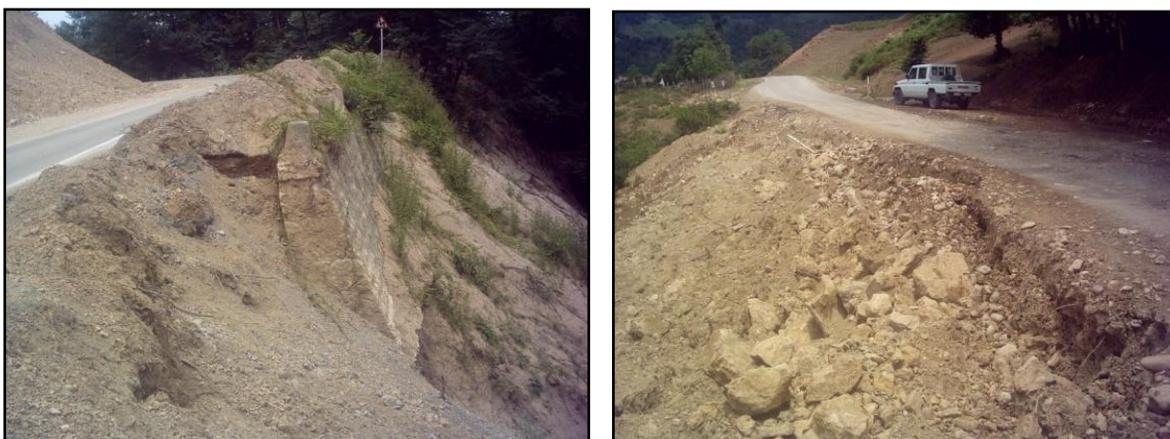
**Fig 1:** Examples of damages caused by landslides in Bandben-Laie road.
